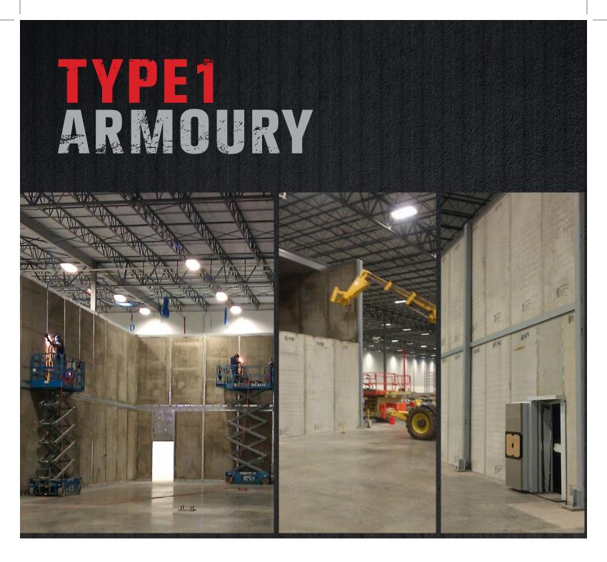
VSA concrete panels are manufactured of a combination of concrete products and security fibres enclosed within a metal frame.
